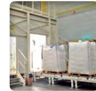
➤ Conveyor and automation
